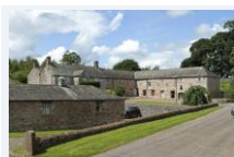
PENRITH Hackthorpe Hall, Hackthorpe
