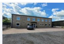
PENRITH Hallin House Offices, North Lakes Business Park
